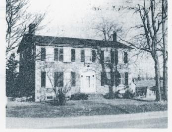
Masonry. Four pilasters flank the side lights. The eliptical wooden fan over the door was used as an alternative to a glass fanlight and is capped by an eliptical cut limestone arch and keystone. The door and brick steps are later replacements.
