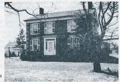
Exterior shutters are a complete set original to this house. Mr. Bean restored them and duplicated the missing set by faithfully copying each of 129 parts. Some windows have had larger glass panes added over the years replacing the original multipaned windows.
